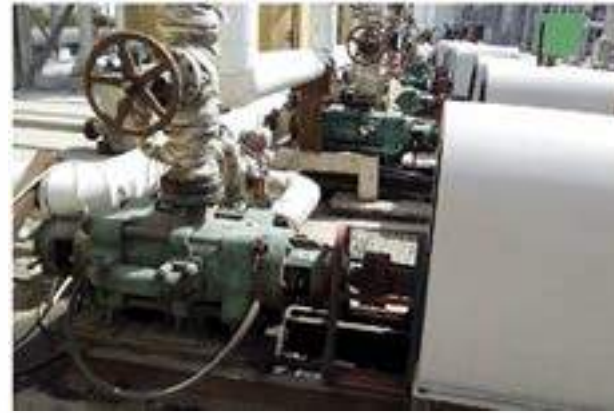
平煤集团联碱厂母液泵应用现场 (型号: ZDF150-30×7 数量: 7台套) Pingmei Group AI factory Mother liquor pump working site (Model: ZDF150-30X7, 7sets.)
