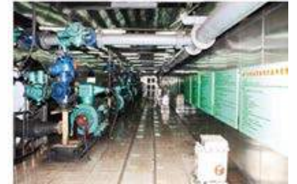
枣庄矿务局 (型号: MD155-67×9, 数量12台) Zaozhuang Cocal Mining Administration (Model: MD155-67×9, 12sets)
