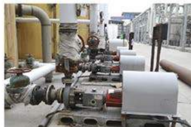
宜化集团化工流程泵应用现场 (型号: ZE300-400 数量: 11台套) Hubei Yihua Group Chemical process pump (Model : ZE300-400, 11 sets)
